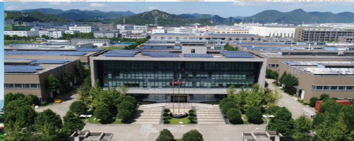
Deli Ningbo Jiangbei Industrial Park
